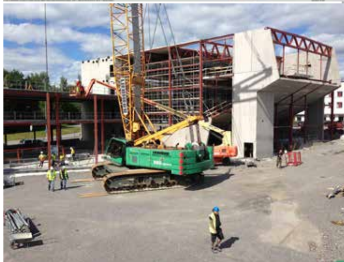
Images: (above) BIM model of prefabricated steel; (middle) Structural BIM model (below) Örebro Business School in construction, Sweden. Images courtesy of Juul Frost Architects
